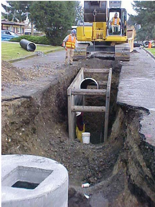
Contractor installs a storm drain pipe on Leschi Road.
